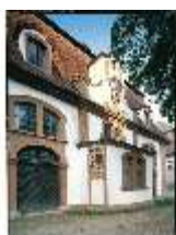
Ell.I, Reithalle, Ostfassade, DE003107, BSV-
